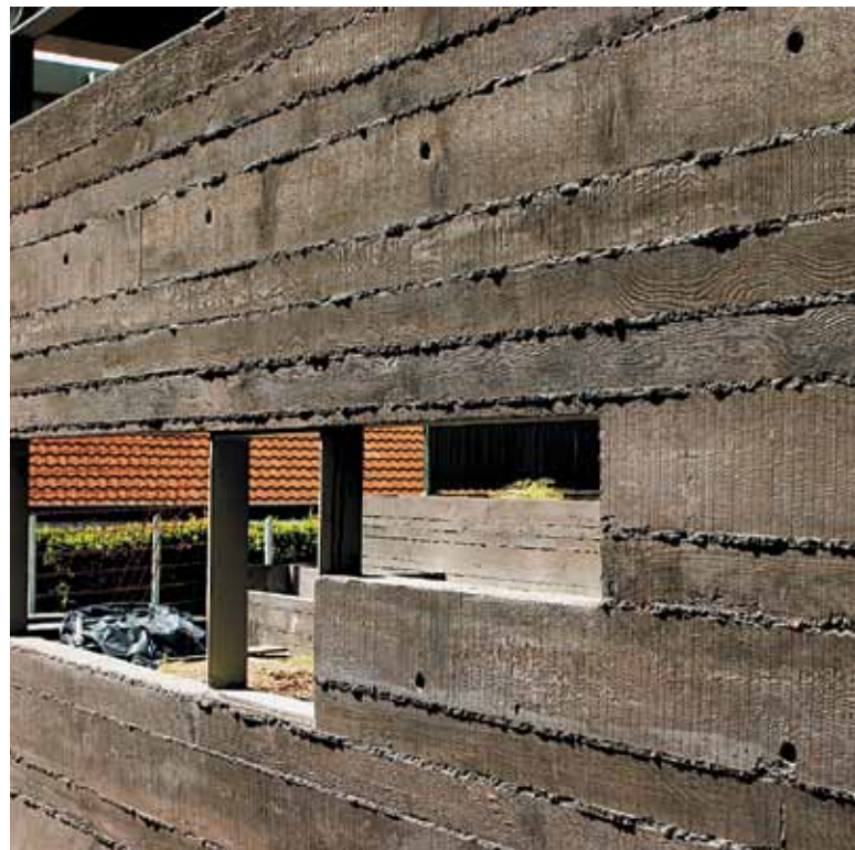
A rustic, natural finish complete with authentic timber texture was created using concrete. Oregon timber was used as the formwork. CCS Panther pigment was used to colour the concrete. Architect: Brian Steenbyk.
