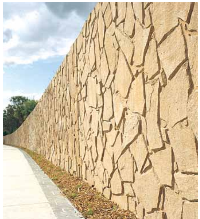
Patterns and textures were embedded into the concrete at the pre-cast concrete plant using specially designed forms and then erected on site. Colour: CCS Honeycomb.
