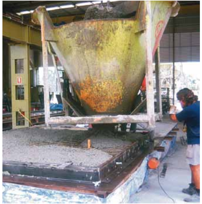
Coloured Concrete being placed into a precast form.
