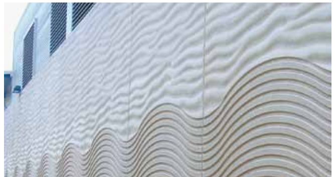
Pre-cast wall at a coastal shopping centre showcases a mixture of texture, achieved with the use of a form liner and shotblasting to emulate sand tracks and ripples.
