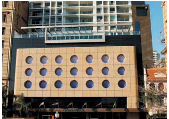
A wonderful example of how a simple but highly effective pre-cast panel design adds character to a building facade. Pre-cast panels coloured with CCS Honeycomb.
