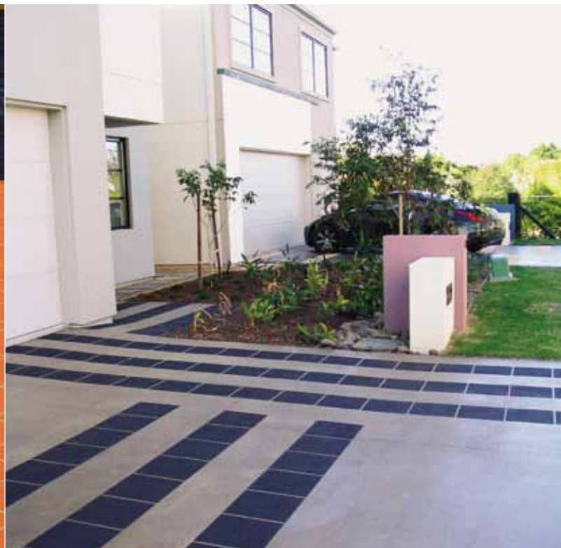
This contemporary driveway has been integrally coloured with CCS Bonsai pigment, then taped in a tile design and coloured with CCS Storm Grey Resurfacing Compound.
